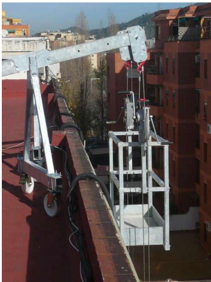
Suspended platform Basic 500 with 2 hoists
