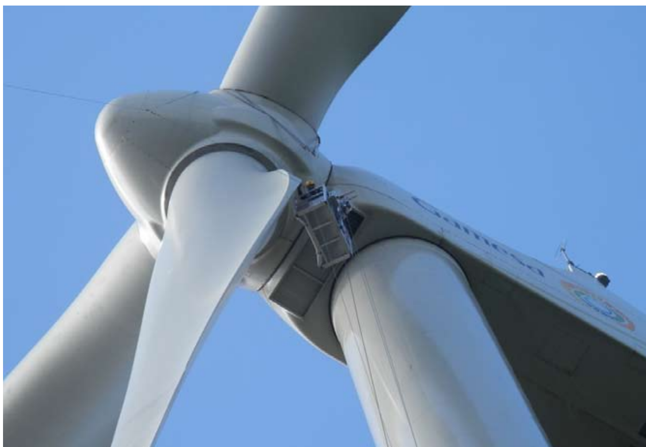
GAMESA G10X, blade maintenance (output edge access)
