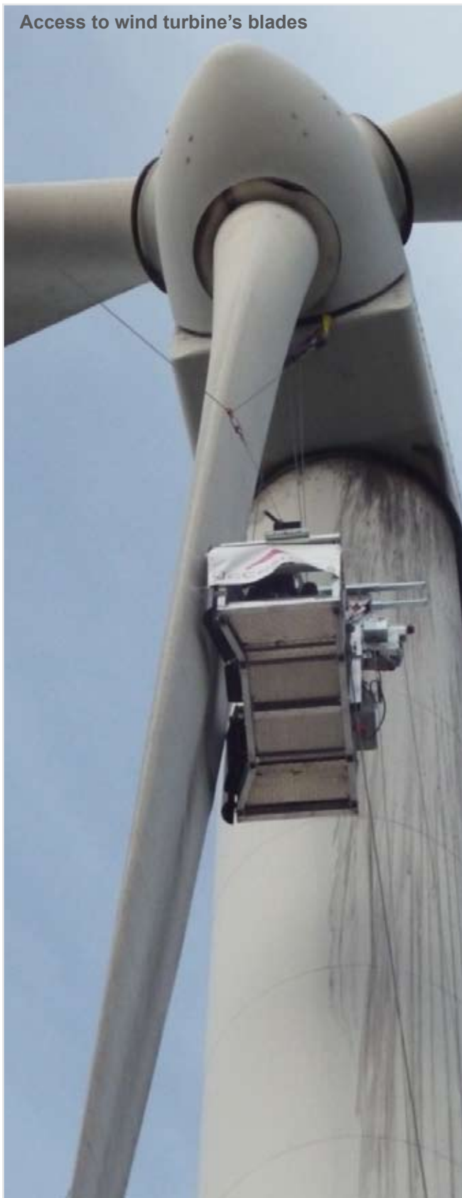
Access to wind turbine's tower
