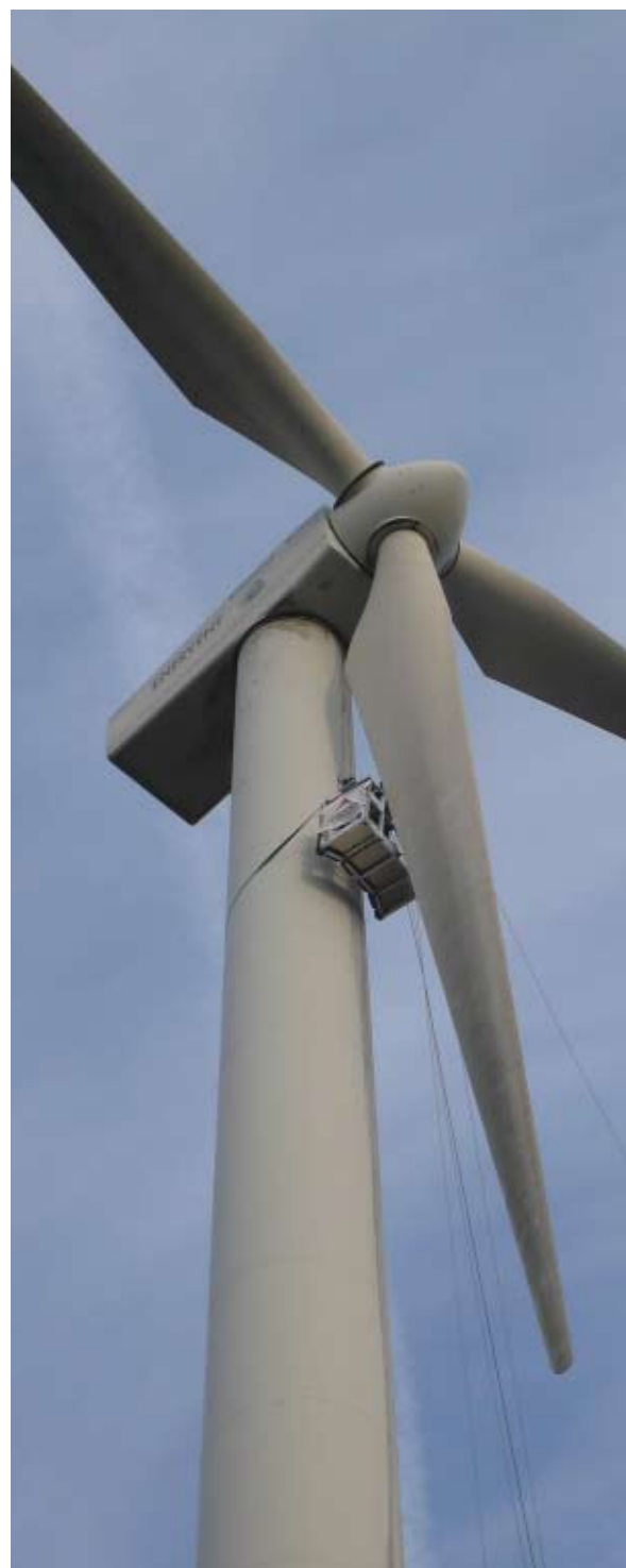
GAMESA G4X y G5X, tower maintenance (cleaning)
