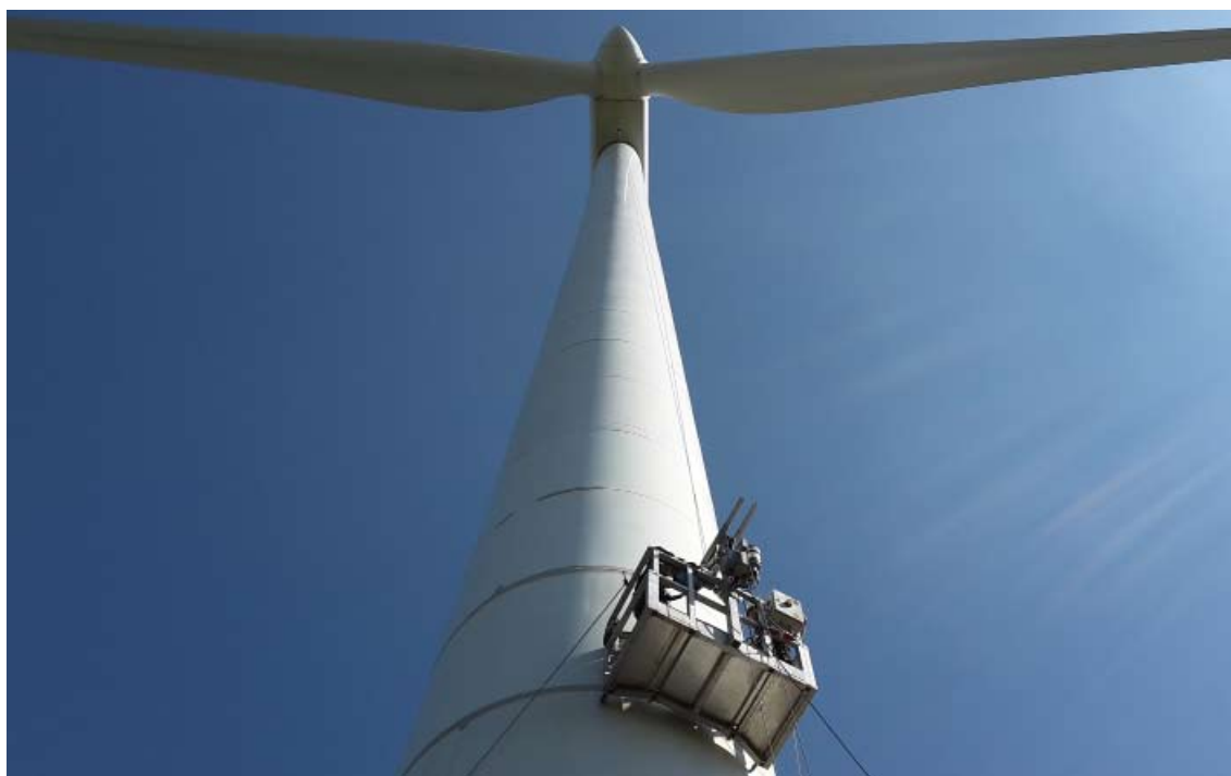
VESTAS V90, tower maintenance (joint repair)
