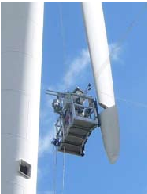
MADE, blade maintenance (end)
