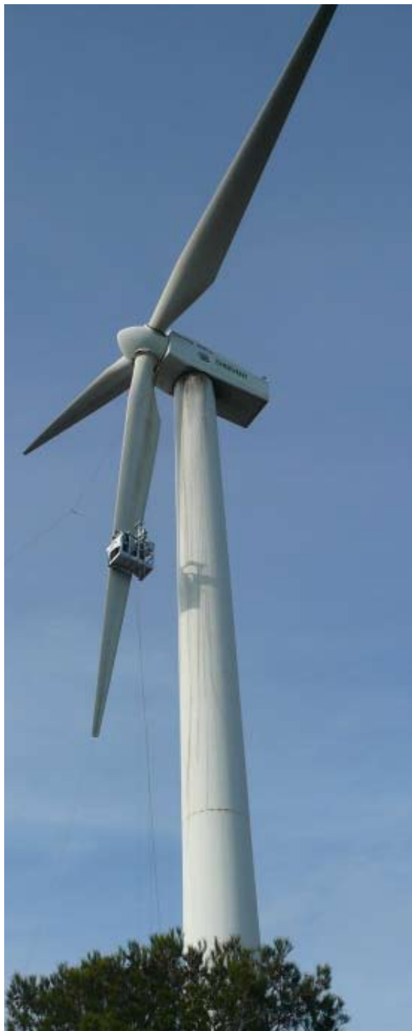
GAMESA G4X y G5X, blade maintenance (fiber)
