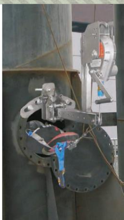
MW manhole rescue arm with ARR.
