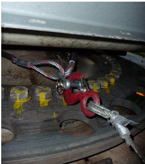
This is the situation when the first wire rope is installed:
