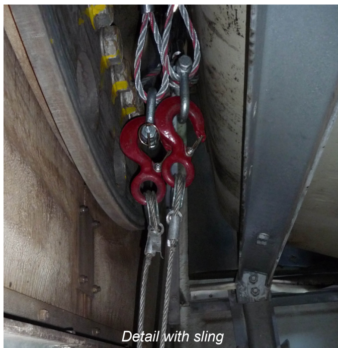
This is the situation when the wire ropes are installed:
