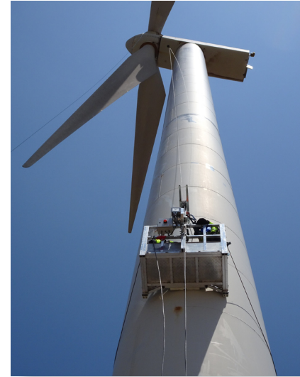
Tower maintenance ( joint repair ).
