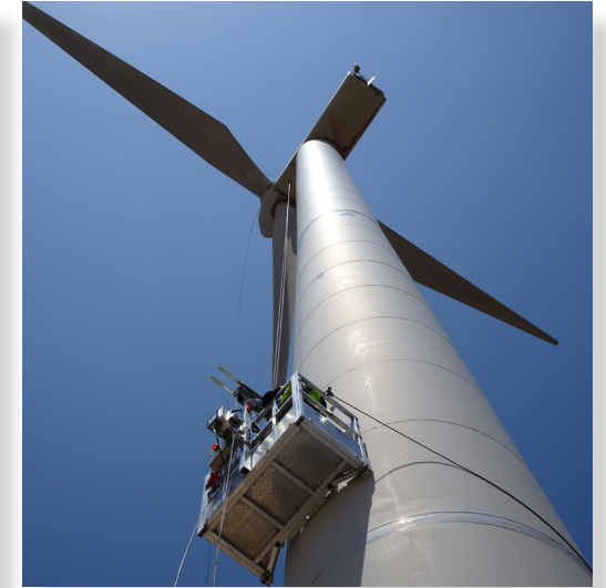
Tower maintenance ( joint repair ).
