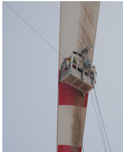
Tower & blade's cleaning works.
