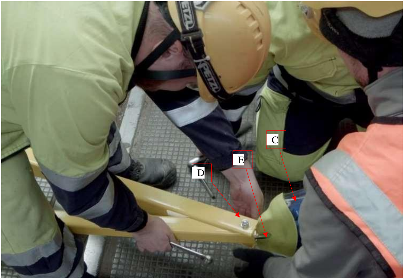
Installation of retractable type fall arrester on rotary arm
