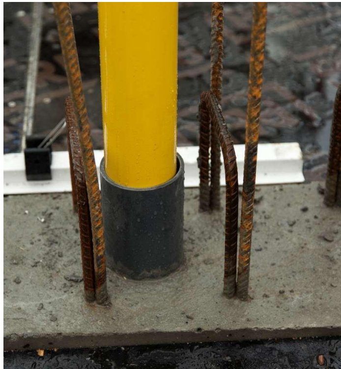
Rotary arm after embedding in socket
