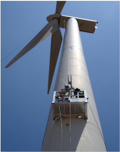
Tower maintenance (joint repair).
