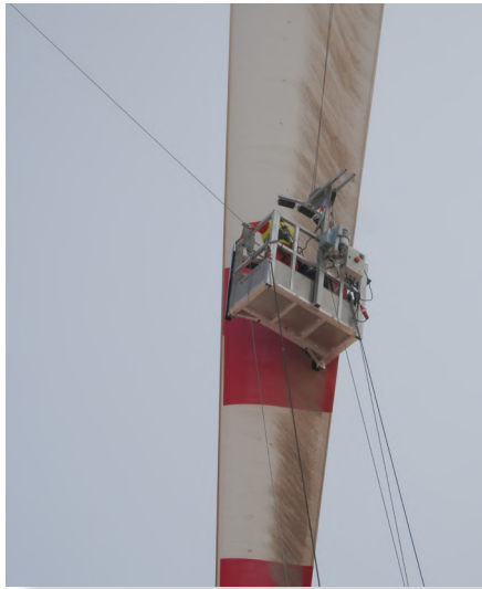
Tower & blade's cleaning works.
