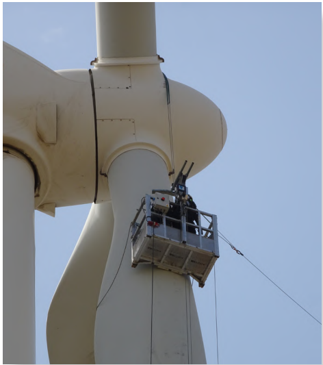
Access to wind turbine's blades and towers for cleaning or maintenance works.
