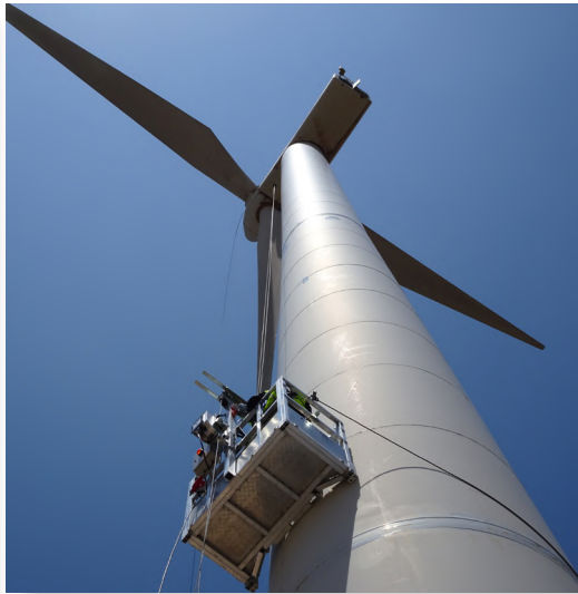
Tower maintenance (joint repair).
