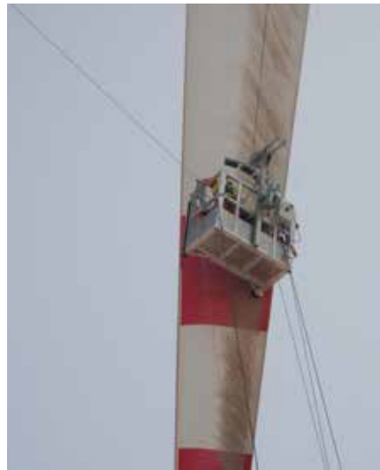
Tower & blade's cleaning works.
