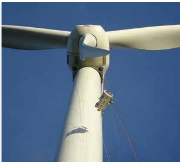
Access to wind turbine's blades and towers for cleaning or maintenance works.
