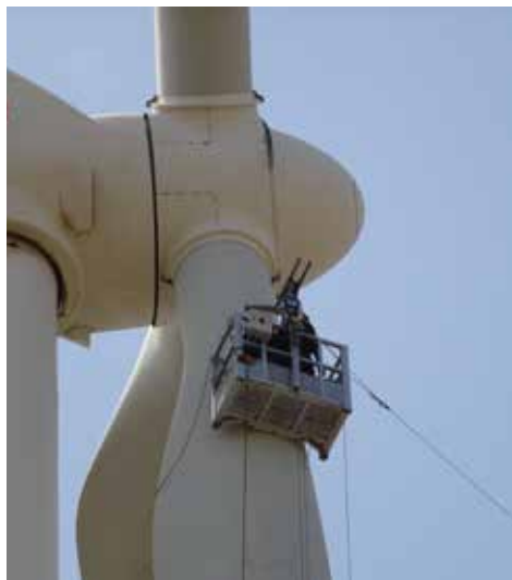
Access to wind turbine's blades and towers for cleaning or maintenance works.
