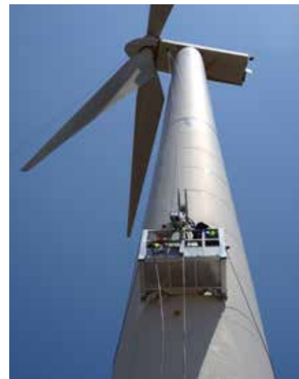
Tower maintenance ( joint repair ).
