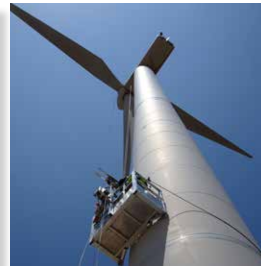
Tower maintenance ( joint repair ).
