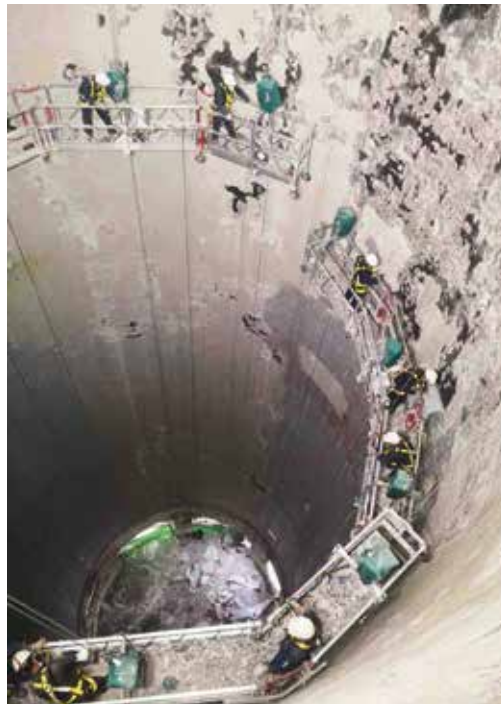
◀ Angular suspended platforms for maintenance inside the silo Design, manufacturing, customer training and assembly of 4 customised suspended platforms and 2 KOMPLET suspended platforms with special beams.
