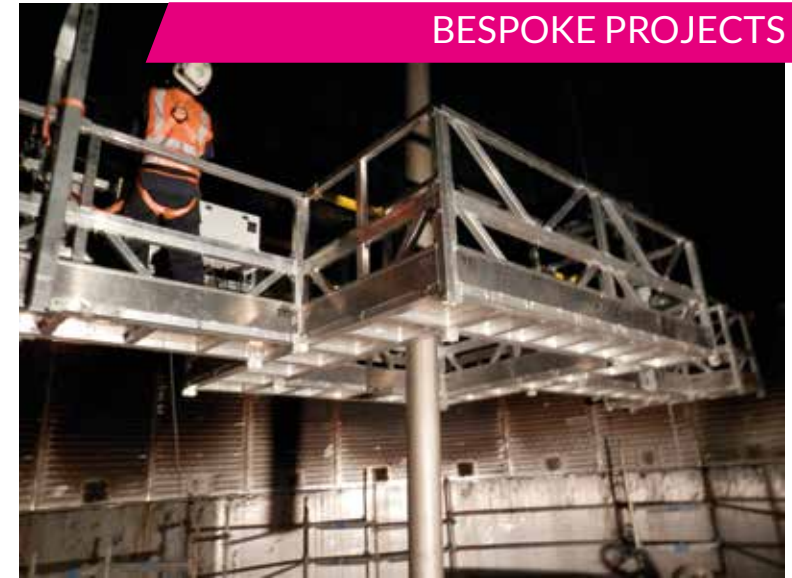
◀ Suspended platforms for construction of designer buildings Double deck platform for construction of ventilated façade and KOMPLET platform with special suspensions for construction of curved buildings.
