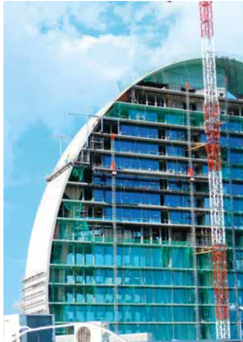
◀ Suspended platforms for construction of designer buildings Double deck platform for construction of ventilated façade and KOMPLET platform with special suspensions for construction of curved buildings.
