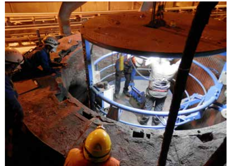
▲ Platform for converter coolant (BOF maintenance) Large-format permanent platform to descend into conduits of more than 60 meters high inside a steel mill.
