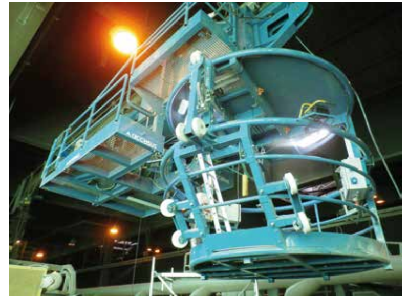
◀ Circular suspension platform for chimney work Circular (pentagonal) suspended platform designed for chimney works.
