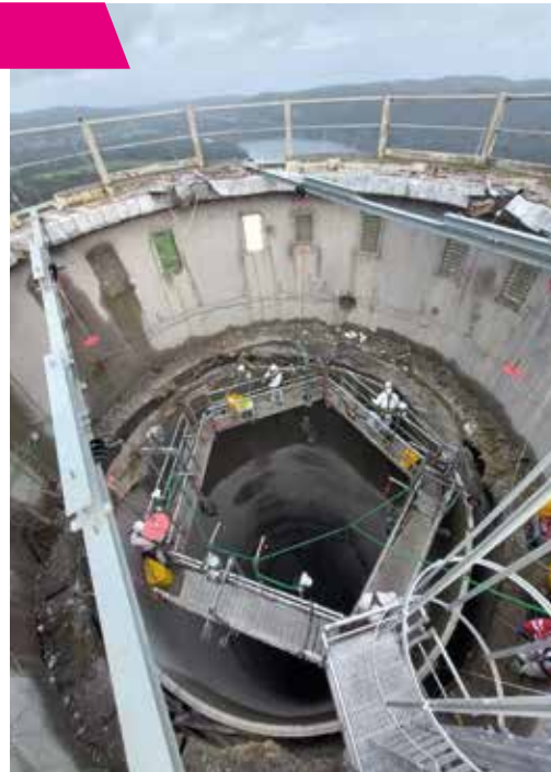
◀ Circular suspension platform for chimney work Circular (pentagonal) suspended platform designed for chimney works.
