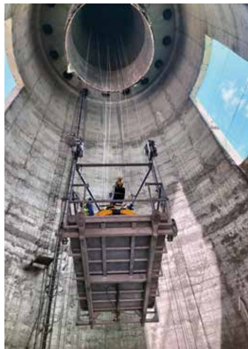
◀ Demolition of a chimney using a suspended platform with a robot Suspended robot platform for chimney demolition.
